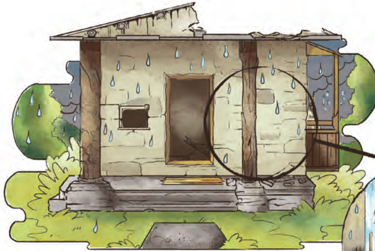
1. Earthquake causing damage to home or granary
